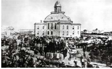
Tarrant County's second courthouse built in 1876-77 and razed in 1894 for the present one to be built.
